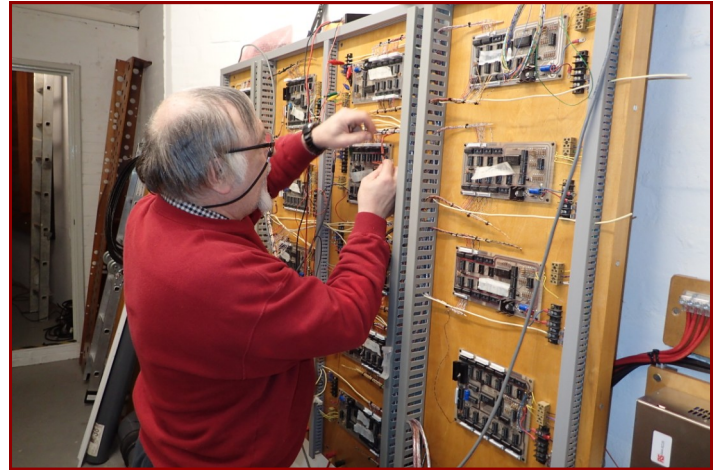
Above: Andrew Barham wiring the relays that link the chamber to the console
